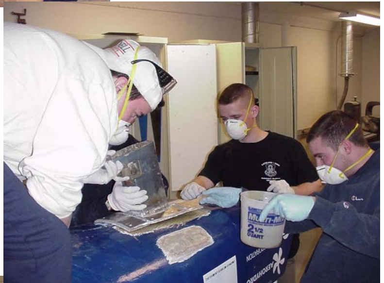
John, Steve and Bob applying roving and resin under mounting flange.
